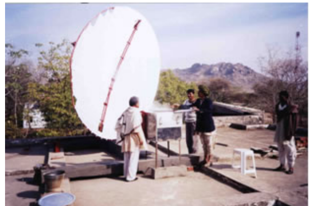
Fig.4 9.7m 2 Scheffler Reflector at the main kitchen of the Barefoot-College in the village Tilonia, Rajasthan, India.
